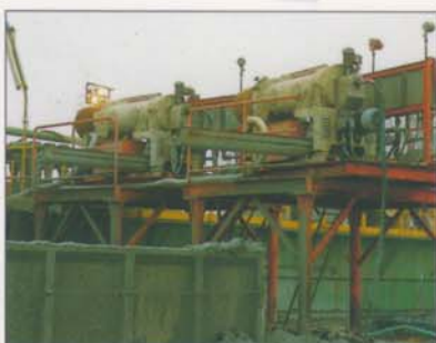
Drilling mud recovery
